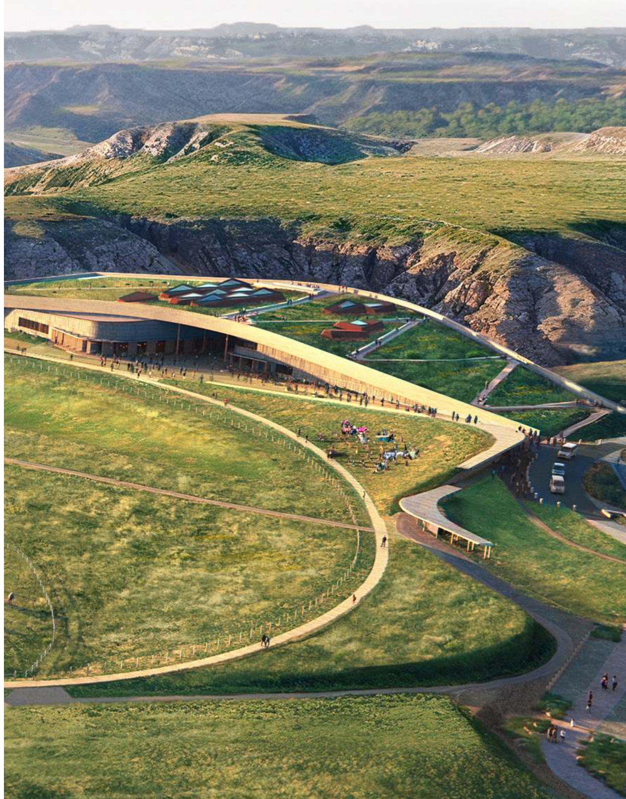
ABOVE: Once the Theodore Roosevelt Presidential Library is completed, it will naturally flow into the native landscape
